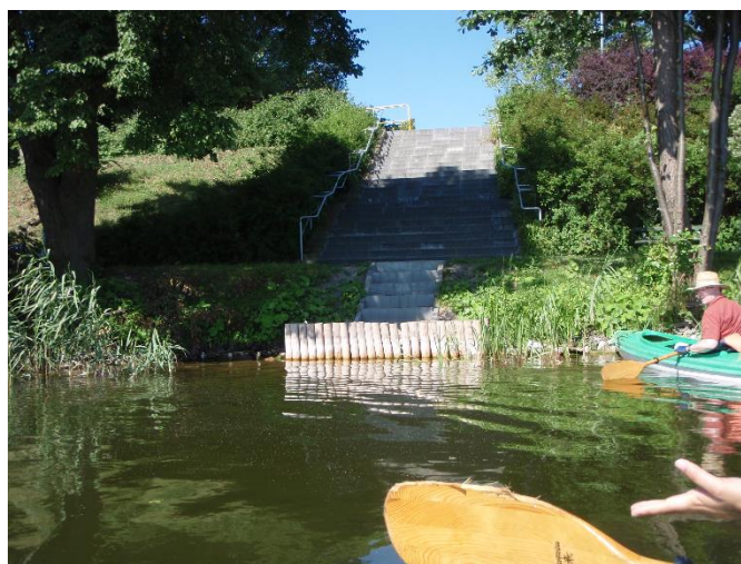
Figure 18: Access point of the lake where sedimentation retention wall has been built
