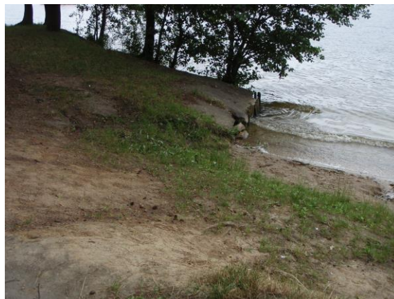
Figure 15: shoreline erosion around along the shoreline
